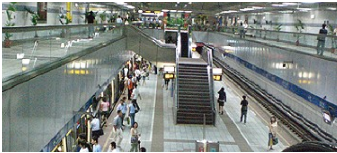
* 120 sets of ST series speed dome cameras are already used in the Taipei MRT stations
